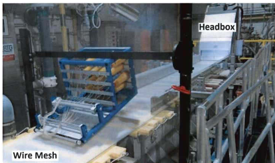
Figure 3-15. Installed feeding frame on the paper machine forming table.
