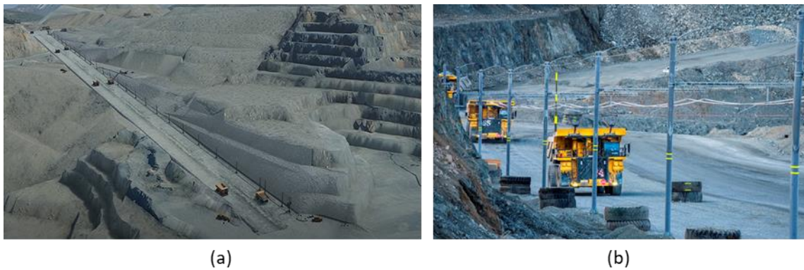
Figure 6. (a) The overall view of trolley-assist system installation at the Copper Mountain mine in B.C., Canada; (b) Haul trucks connected to the trolley-assist system network in action at the Copper Mountain mine [68].
