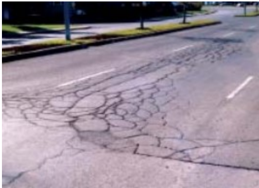
Figure 13 – Fissure en carrelage (MTQ, 2011)
