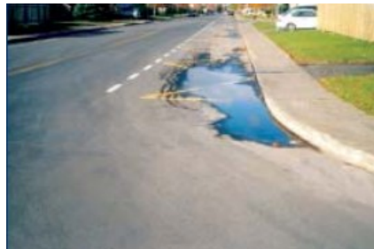
Figure 16 – Affaissement (MTQ, 2011)
