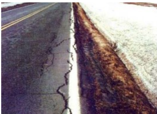
Figure 13 – Fissure en carrelage (MTQ, 2011)
