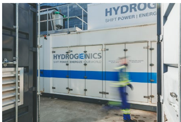
Figure 23 : 1.2 MW electrolyzer manufactured by Hydrogenics (now Accelera by Cummins). Credit: Harnois Énergies.
