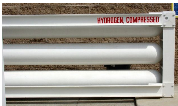
Figure 22 : Stationary hydrogen storage using Type I tubes [167].
